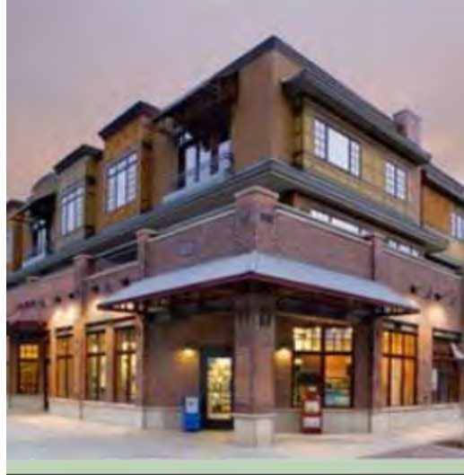
Figure 8 Mixed Use Building Architectural interest achieved through a mix of building materials, overhangs, offsets and cornice treatment.
