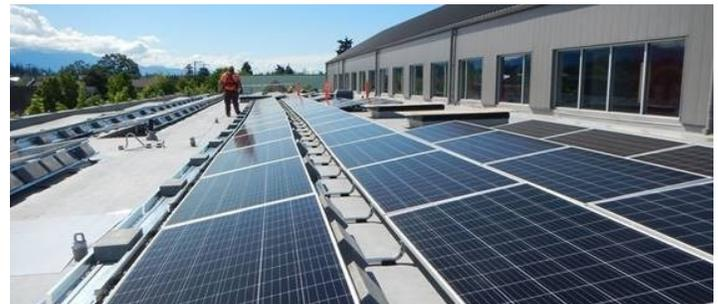
The installation of 132 solar panels on the roof of the Sequim Civic Center is complete. The panels were connected to the City’s utility grid on May 27 and are now generating energy.
